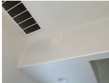
Interior sheetrock patchwork around walls
