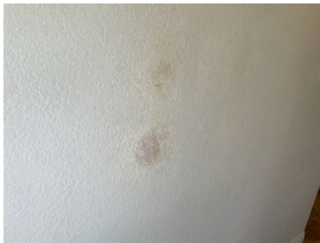
Interior sheetrock patchwork around walls
